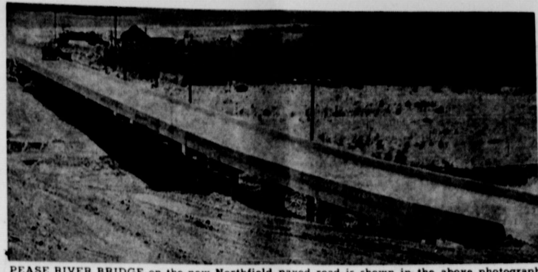
PEASE RIVER BRIDGE on the new Northfield paved road is shown in the above photograph. Modern concrete structure replaces the old wooden bridge which was frequently in poor repair. The new bridge is of the latest design and cost of construction was the largest item on the new highway. The new bridge is located at the point from which the former wooden bridge was removed, but the approach from Northfield was changed which removed sharp curves and shortened the route.—Photo and engraving courtesy Childress Index.
