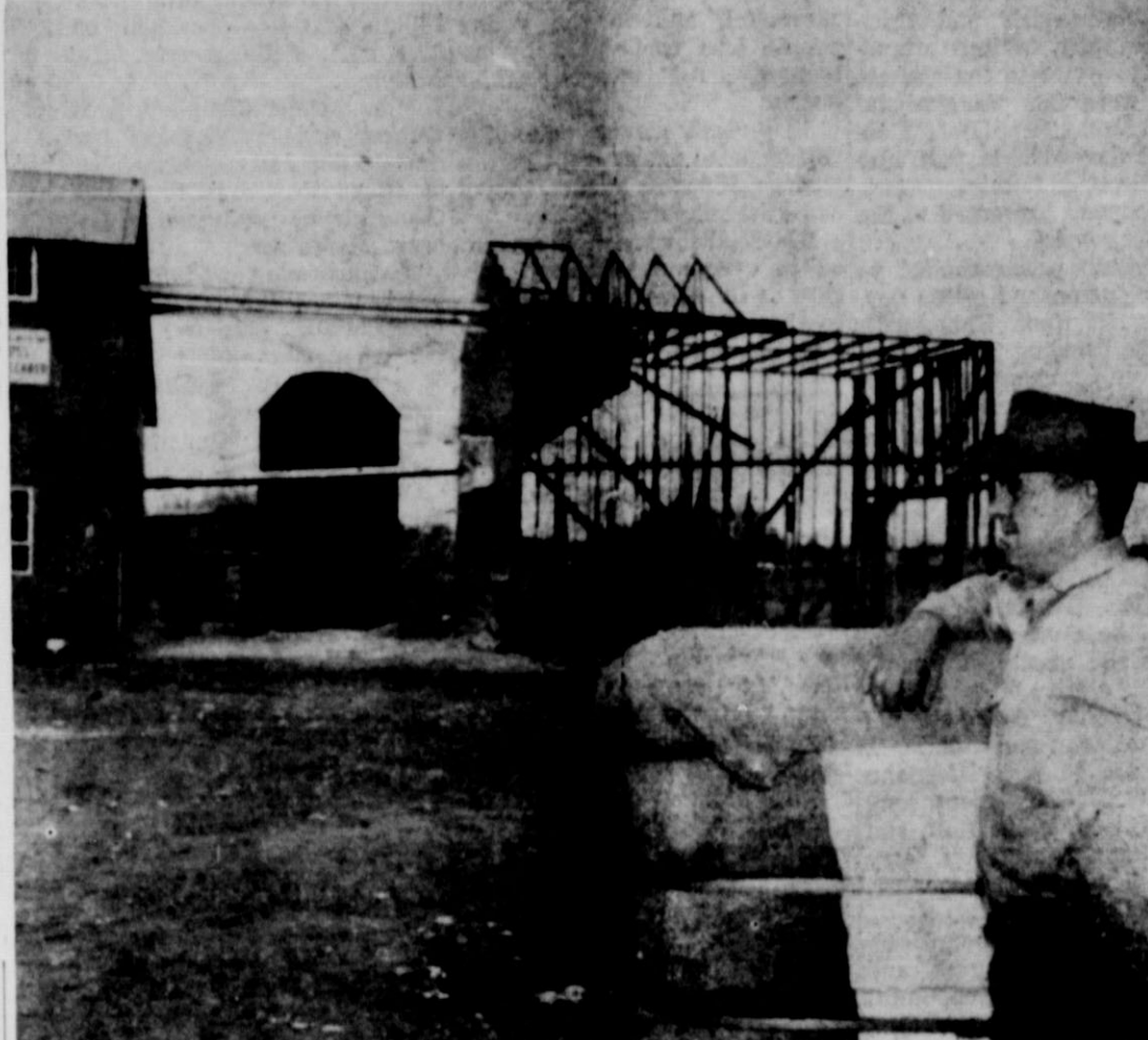
LONG SILENCE—West Texas Gin manager Bonnie Keltz looks at the plant seed house being dismantled (in background; now completely removed) as work is started to move the gin to a new site on State Highway 70 about one mile northwest of town. At the time this picture was made one of the last bales of the 1960 season was being ginned. Familiar musical hum will be silenced permanently when the final bale is ginned and the last gin in Matador is moved. From one to three gins have operated here for about 60 years. West Texas is building a more modern plant on a site of about 11 acres purchased from R. E. Campbell Sr. The new site will be more accessible to cotton-growers of the area.
