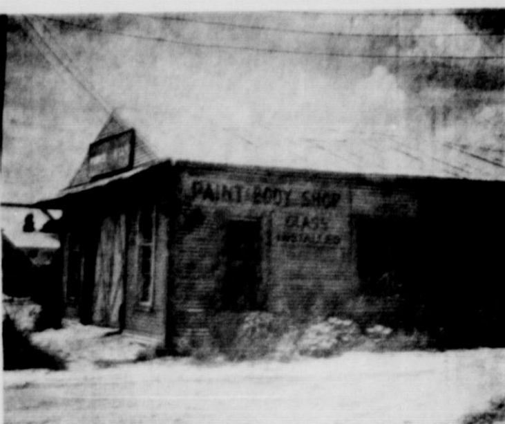
THE TRIBUNE was spawned in this building still standing in Roaring Springs, but soon to be removed.
