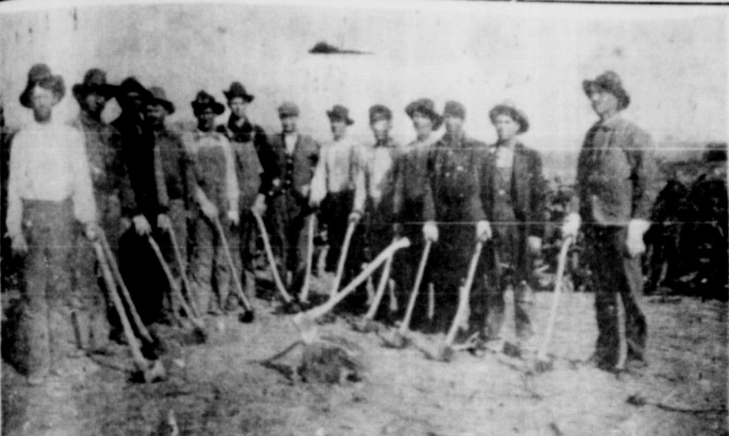
A PLACE TO BUILD A CITY —These workmen are clearing the land to build Roaring Springs in 1913. The names of seven are known. Reading from left to right, No. 1 is Crawford Snow, No. 2 is Jim Cloyd, No. 3 is Walter Carpenter, No. 4 is Jim Swearingen, No. 7 is Nelson Pender and No. 12 is Oscar Calloway. This photo courtesy of C. E. (Tib) Harris. Another print of this picture, belonging to Brooks Calloway, was used last year.
