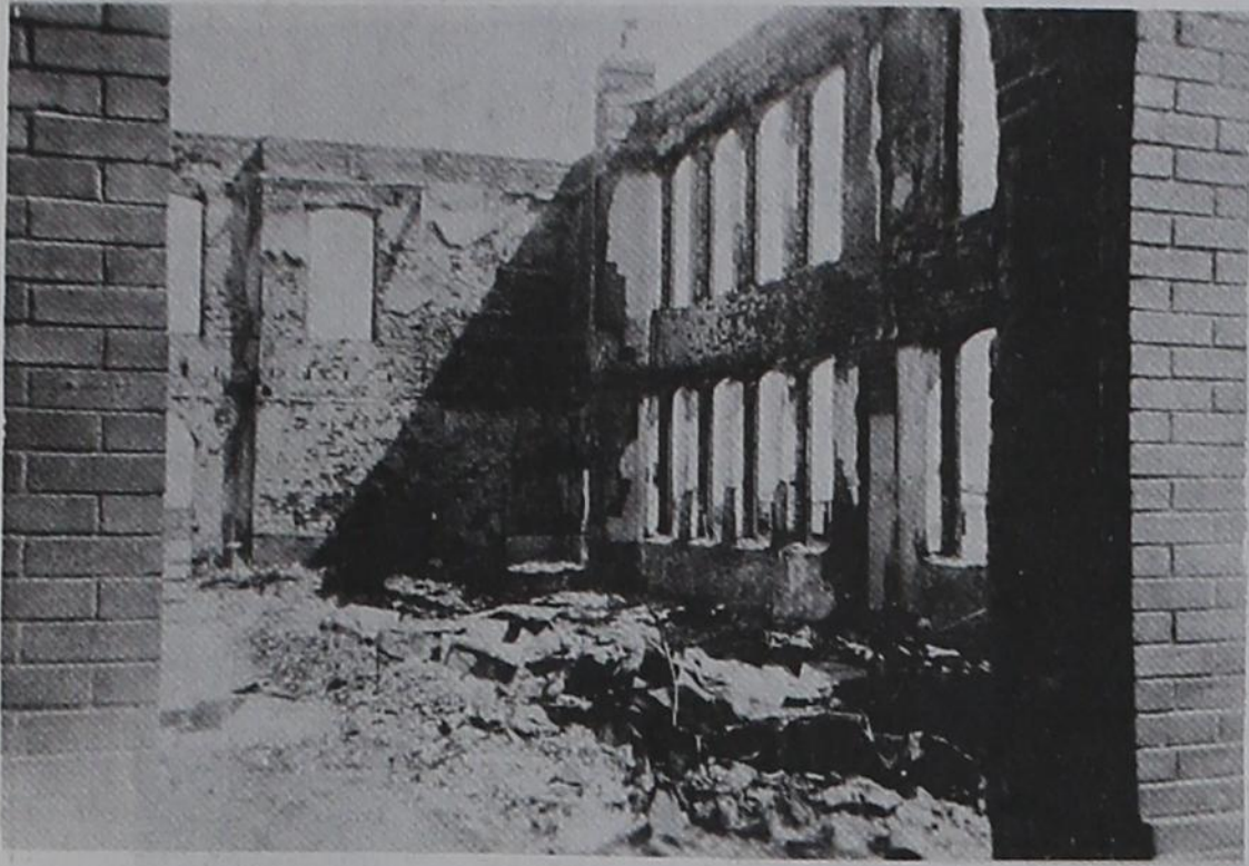
The 3 story brick school building in Roaring Springs burned in 1945.
