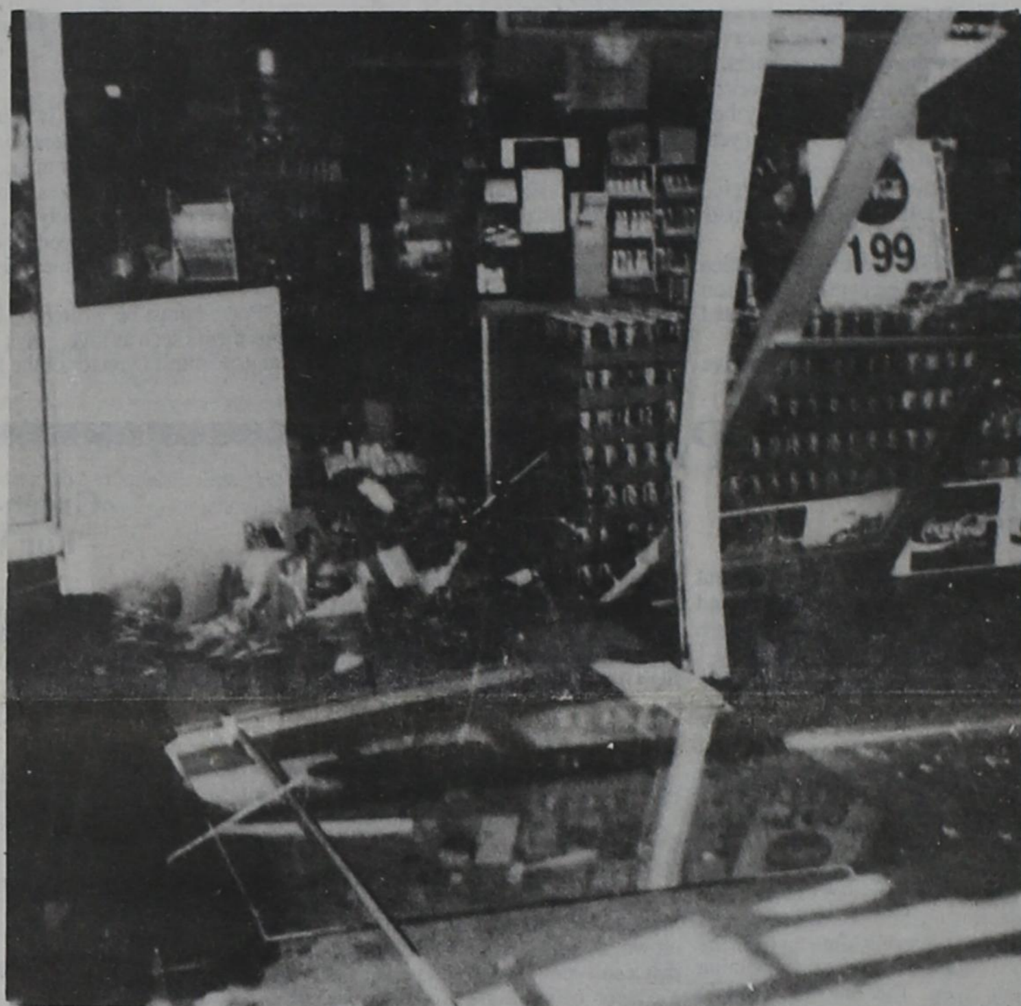
The front windows of the Allsup's Convenience Store on Hwy. 70 in Matador were crashed in when Motley County resident, Cody Barclay, was pulling up in front of the store and lost control of his brakes, Tuesday morning. No one was injured. The store remained open, while workers cleared away the debris. Estimated damages were unknown at newstime.
