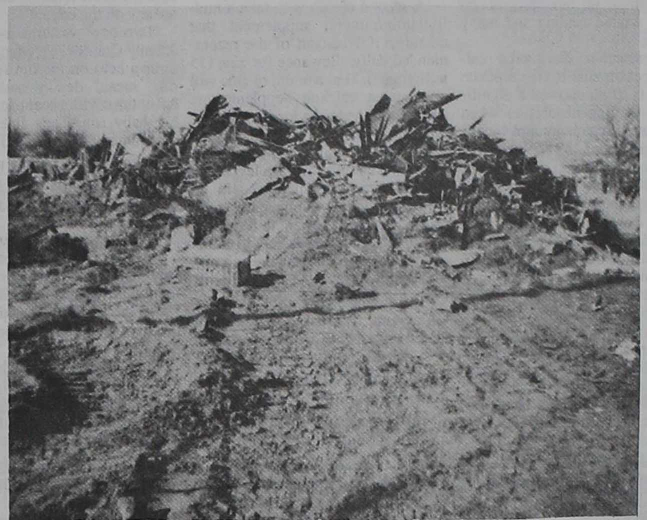
CITY CLEAN-UP — This rubble is formerly the old Westmorland home place. This property was previously owned by John Burnett who recently gave it to the Matador Assembly of God Church. It is north of the present Church building on the corner of Bundy & Newlan Streets.
