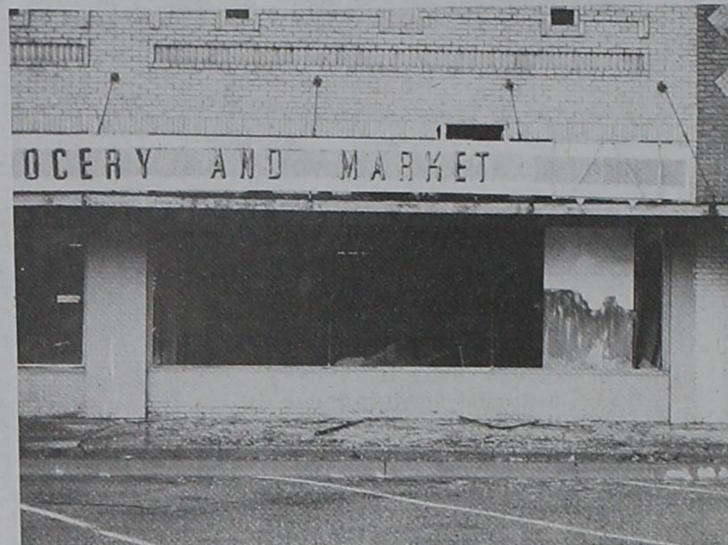
BROKEN WINDOWS — Saturday's storm blew in through the back of the old Spot Cash Grocery building and blew out the big front glass windows.
