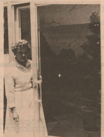
VANDALISM: Motley County Clerk, Lucretia Campbell, is standing at the front door of the Courthouse, which was broken when a large rock was thrown into the glass. The arrow points to the broken glass. The front door of the First State Bank was also broken in the same manner. The courthouse door was noticed on Saturday morning, when election Judges came in to begin the local election. Bank President, Roy Hobbs found the broken glass at the bank around 9:30 a.m. Saturday morning. According to Sheriff Alton Marshall it is suspected that these doors were smashed by the same vandals.
