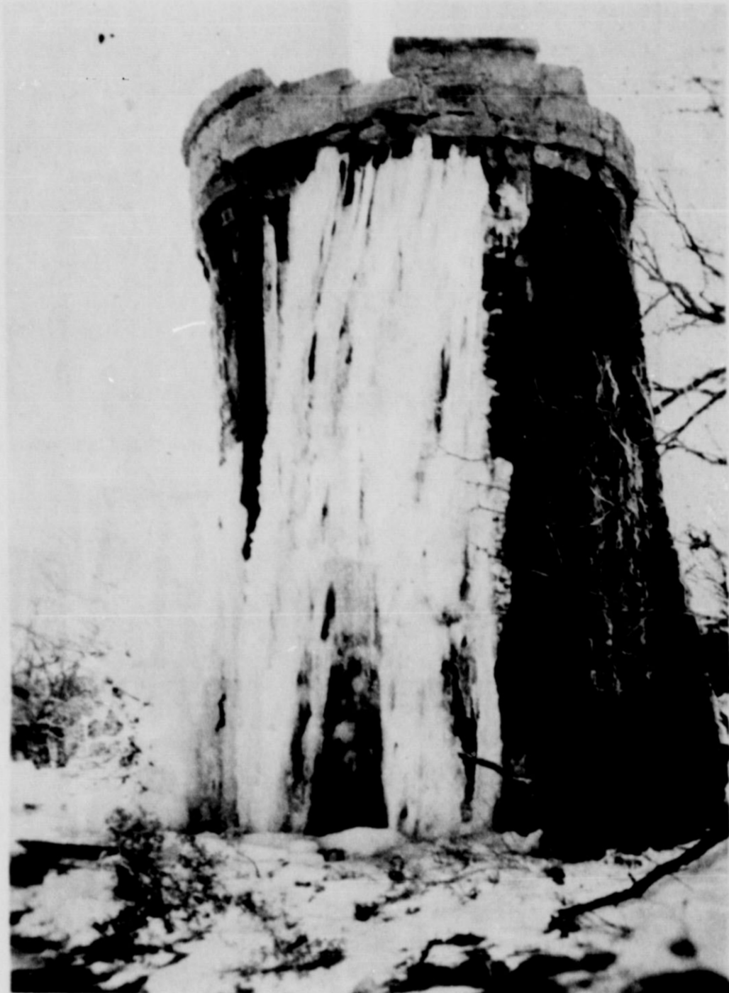
Water Reservoir at Matador Ranch Headquarters Built by the Scots about 50 years ago
