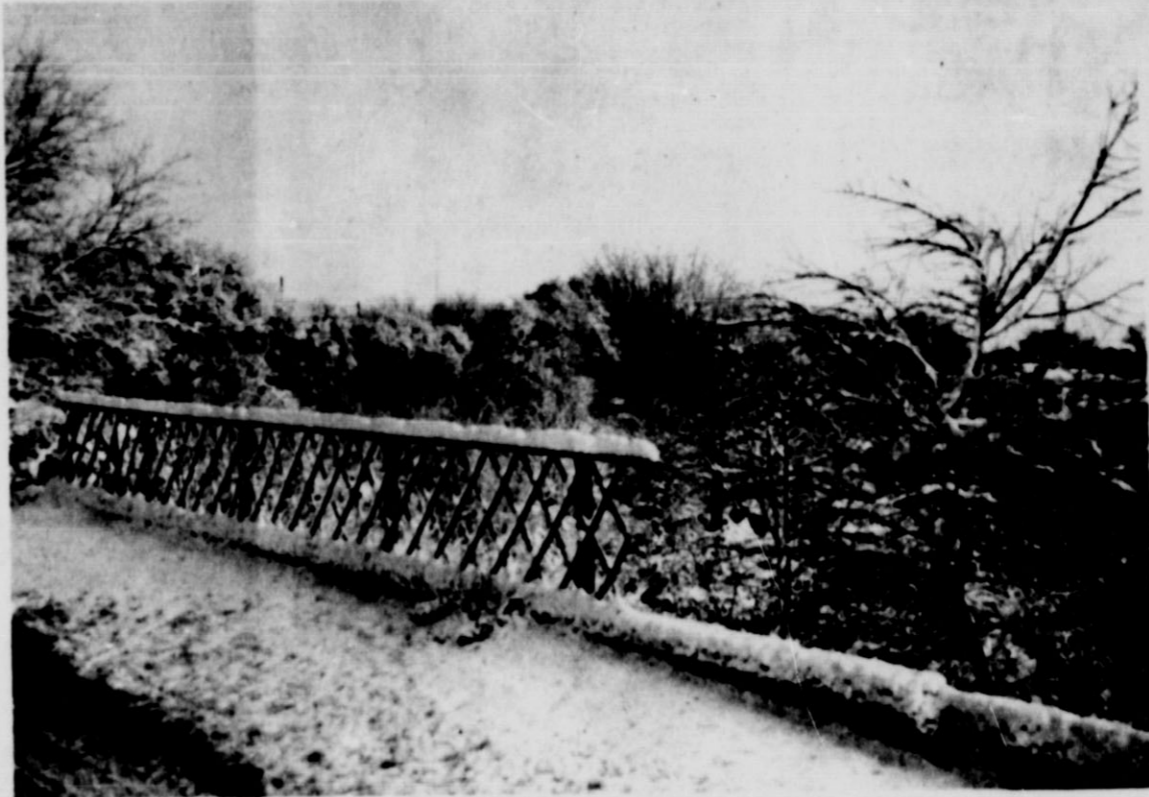
OLD BALLARD CREEK BRIDGE, North Main Street, Matador
