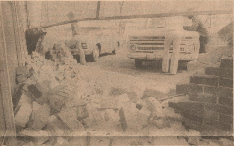
THE WALL CAME TUMBLIN' - From inside the Matador Red X Store, the damage of the Thursday afternoon accident can be seen. Outside, Sheriff Alton Marshall is questioning Melvin Moore, driver of the pickup which hit the store's front. The 1965 Chevrolet pickup, with surprisingly little damage, can also be seen. (Photo by Mary Renfro)
