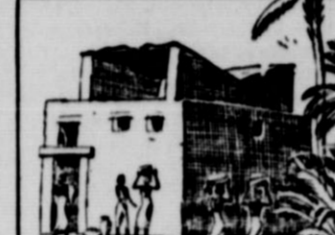
Air Conditioning 2,000 Years Ago. Above—Chariot Tent, Used 1,500 Years Before The "Covered Wagon."
