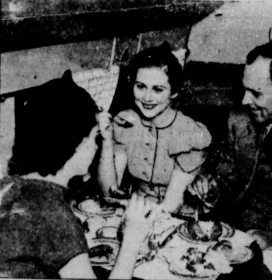
The same feature of excellent meals, which has been a watchword in the past with Transcontinental & Western Air, Inc. of course will be continued on its new Skysleepers. Fried chicken, baked potatoes, salad, and so on, go to make the meal served these passengers...
