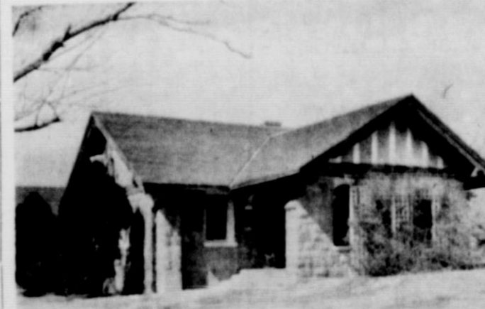
HISTORIC Matador Ranch Headquarters house, one mile southwest of Matador, will be open to the public, 10 to 12 a.m. Friday, (August 5) and 10 to 12 a.m. and 2 to 4 p.m., Saturday, (August 6). The large house was built about 1918, from native stone quarried on the site.
