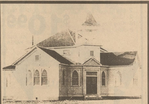
Flomot First Baptist Church Dedicated March 10, 11, 1917. Existing building erected in 1959.
