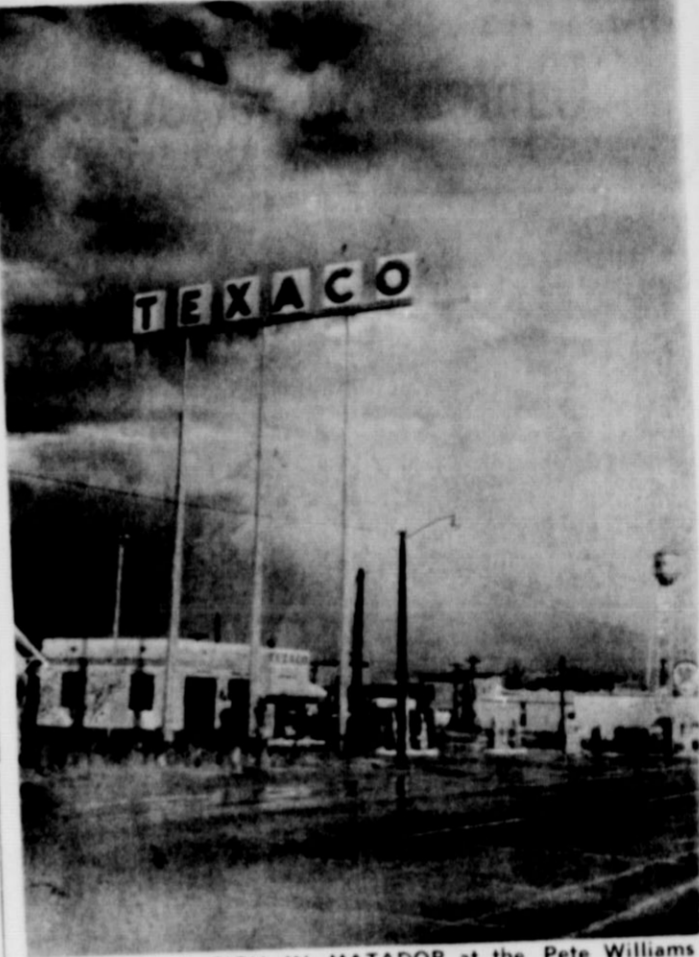
HIGH RISE SIGN IN MATADOR at the Pete Williams Texaco station. The sign was erected two weeks ago during freezing weather. It is 50 feet from the ground to the base of sign and the letters are eight feet high. The sign can be seen from five miles both east and west of Matador on US Highway 70.
