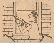
Caulk around doors and windows
