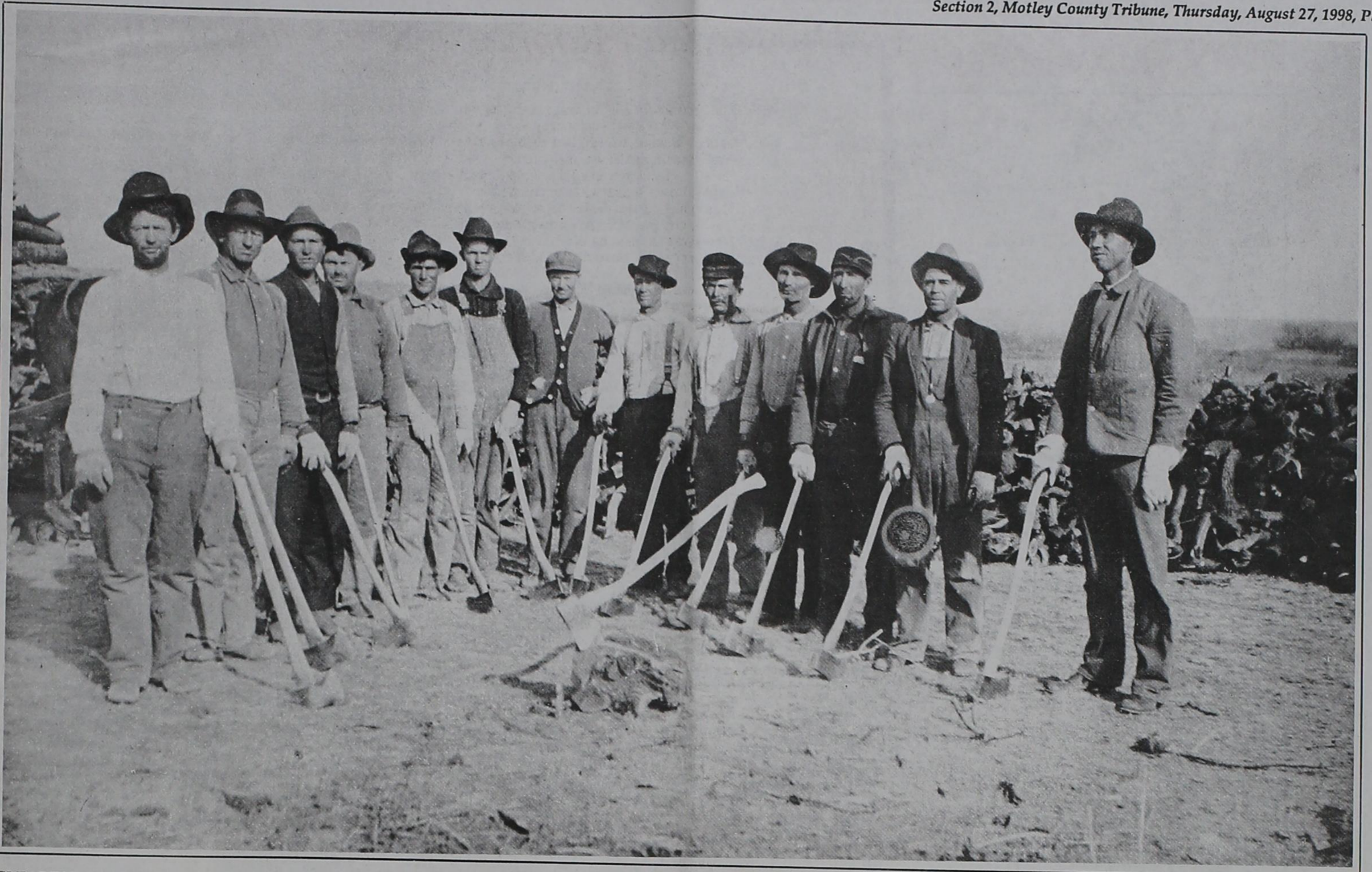
CLEARING THE GROUND TO BUILD A CITY — This photograph was made in 1913, and shows the group of men who cleared the townsite of Roaring Springs. Men in photograph, are from left to right:
