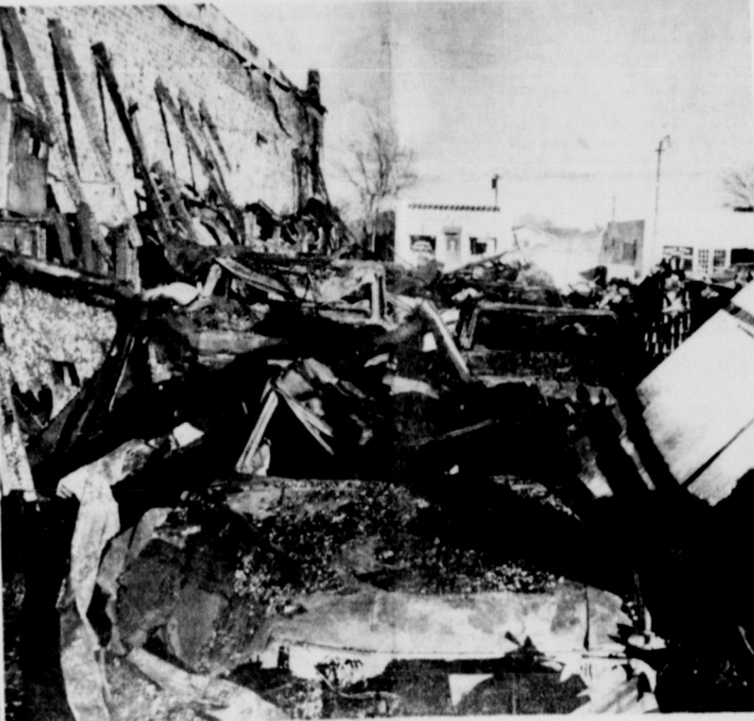
DONE TO A CRISP —New Mercury and Ford automobiles and pickups destroyed in the early morning fire which swept Matador Auto Co. storage building Thursday. Main brick building of the pioneer firm is shown at left. Photo made from point looking toward Main Street. —Tribune photo
