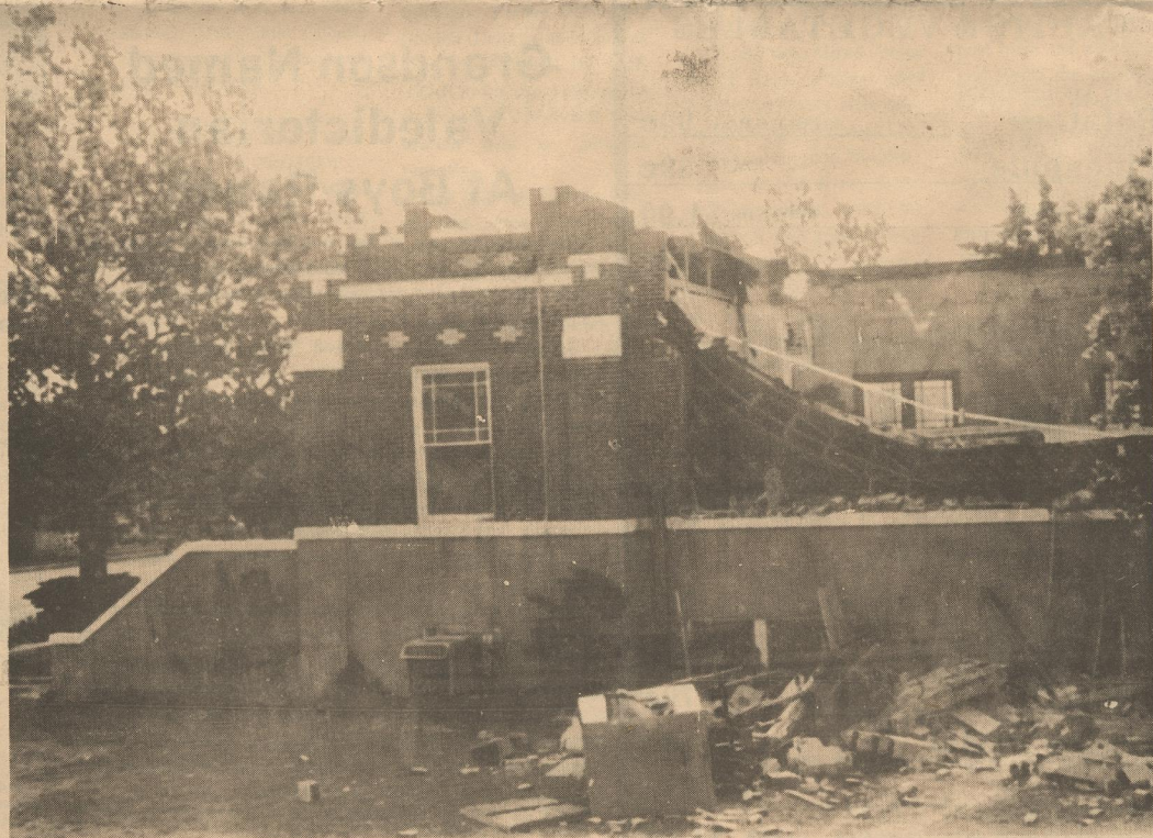
First United Methodist Church, Matador, Following Collapse of the Roof, Wednesday.
