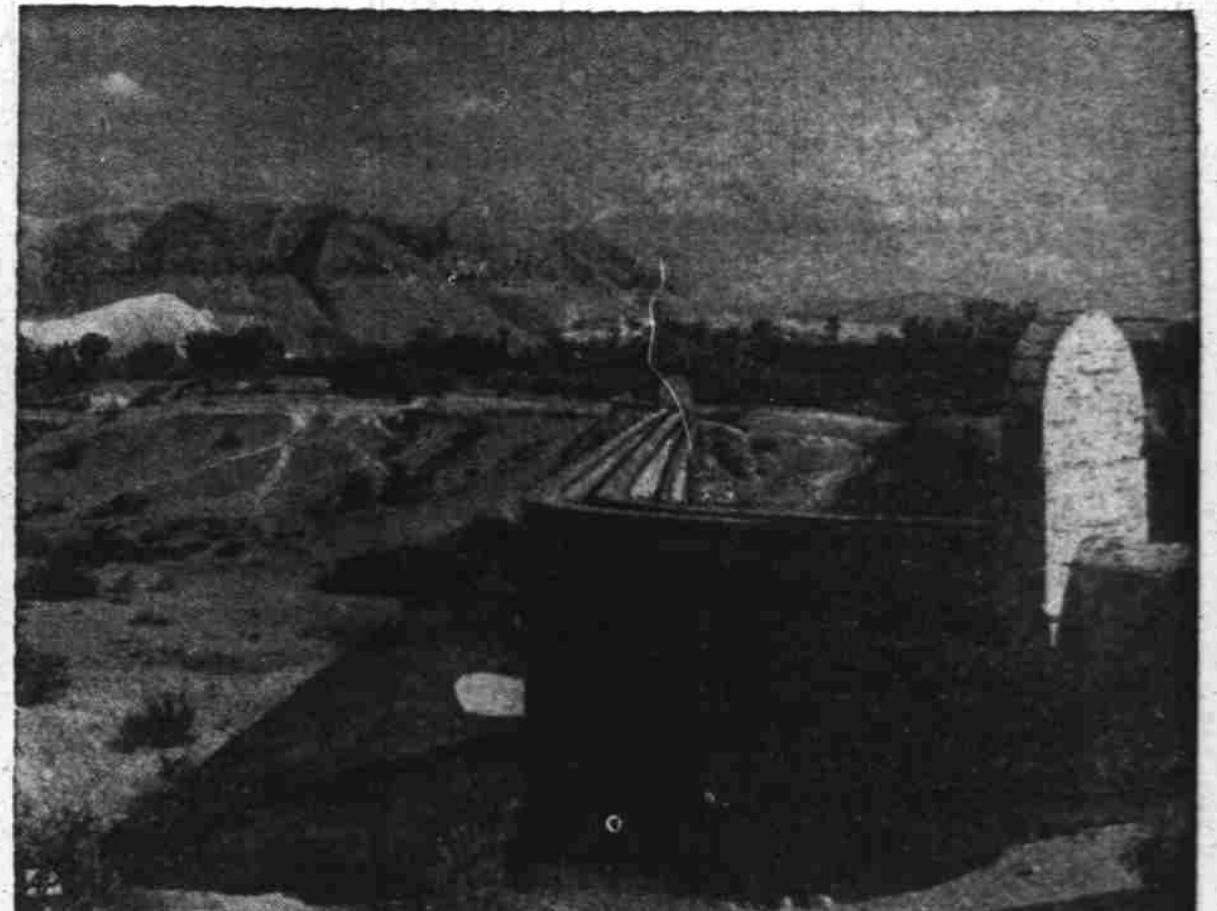
ARABIAN FLUME — A bridged irrigation flume carries waters of the Spring of Elisha to Arab banana plantations near Jericho. Mount of Temptation is in the background.
