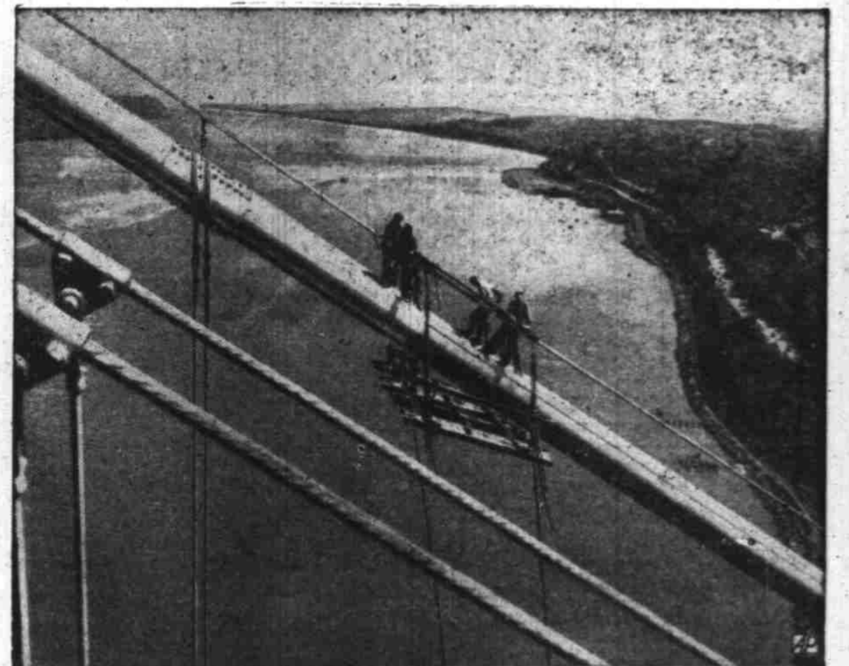
BIG PAINT JOB —A crew works 600 feet above the water at painting the mile-long George Washington bridge across the Hudson river at New York. The job will take four years.
