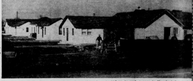
HOUSING PROJECT—Oil and gas exploration activity has stepped up to such a pace in Hansford County that retired rancher has built 10 houses that will be rented to oil field workers. Called the Matthews Addition, cost more than $50,000.
