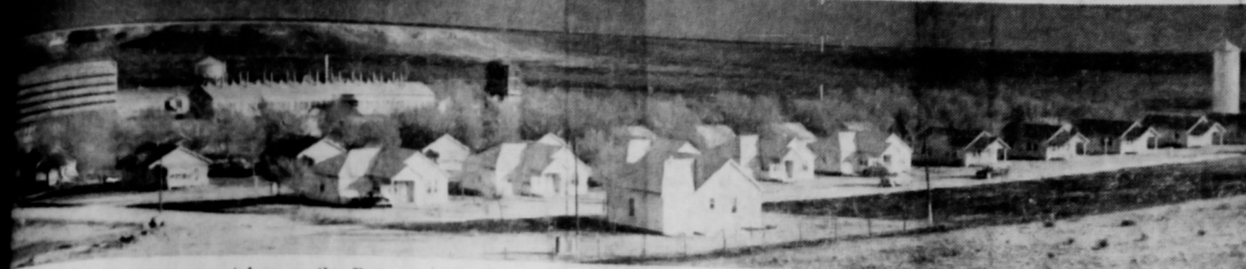
Picture of the Panhandle Pipe Line Commission Station. The picture was taken on the East side of the Station. The Station is twenty two miles North and four miles West of Spearman. It is a quarter of a mile from the Oklahoma State line. It is surprising at the people in Spearman who don't know that a Station like this is even in their county! The people out that way are wonderful. Drive out and visit them some time.
