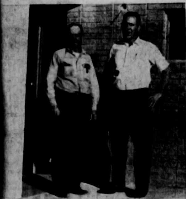
Tractor E. D. Mundy man Hospital Clinic in January building and Dr. H. B. 1964. moved into the new Spear-
