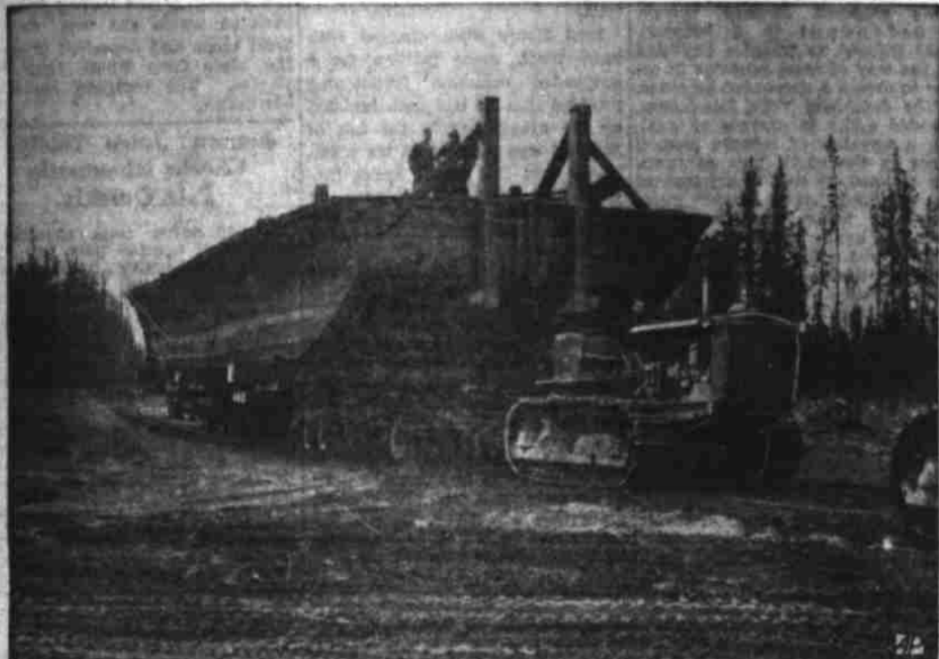
CANADIAN PORTAGE —Powerful tractors haul a 65-ton barge from Fitzgerald, Alberta, to Fort Smith, N.W.T., Canada, for use in transporting supplies for the Canol oil pipeline project.
