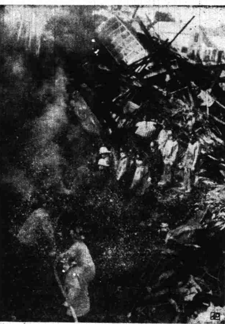
FIREMEN SEARCH BLAST WRECKAGE—Firemen search for victims of a warehouse apartment building destroyed in Santa Barbara, Calif., by an explosion. At least five bodies were recovered from the ruins. Five other persons were injured.
