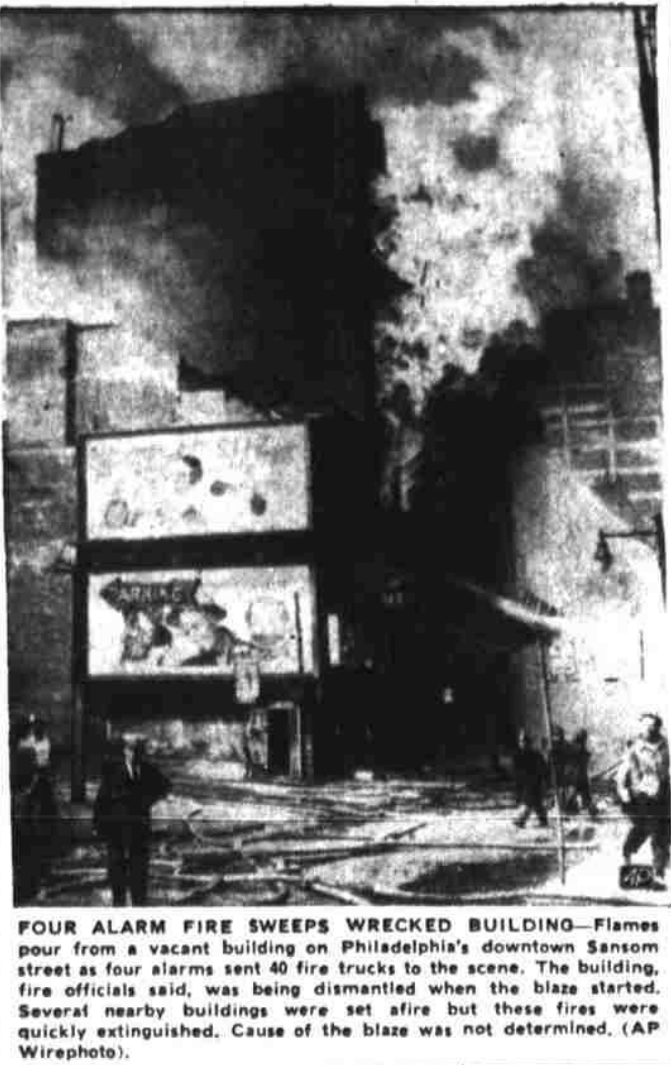
FOUR ALARM FIRE SWEEPS WRECKED BUILDING—Flames pour from a vacant building on Philadelphia's downtown Sansom street as four alarms sent 40 fire trucks to the scene. The building, fire officials said, was being dismantled when the blaze started. Several nearby buildings were set afire but these fires were quickly extinguished. Cause of the blaze was not determined. (AP Wirephoto).
