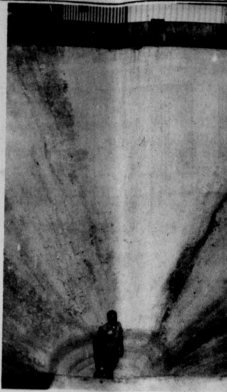
4-Tex Grain Co. is presently enlarging their grain storage facility south of Spearman. Gerald Johnson, elevator superintendent is shown here in the storage pit which will double the capacity of the elevator.
