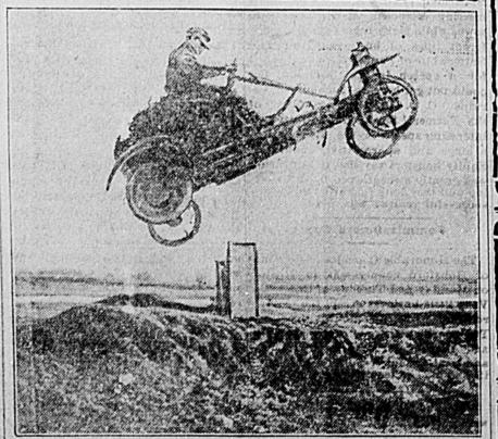
gineer, makes it possible for any light car to reap through the air over obstructions. The device in the rear of the machine does the trick. The photo shows a test car, equipped with the Gauthier device, making a high leap in Paris recently. The device is controlled from the chauffeur's seat.
