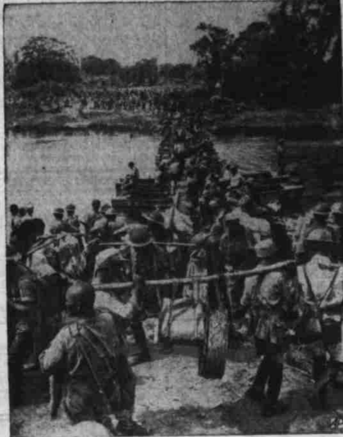
BURMA ADVANCE —American and Chinese troops cross an improvised bridge, built of planks, boats and empty gasoline cans, over the Mogaung River during the Burma campaign.
