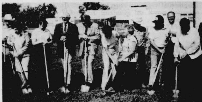
A scene from the groundbreaking held Monday, June 13 at the Stationmaster's House Museum. Pictured above are Johnny Lee, Joyce Johnson, Ann Cluck, J.C.
