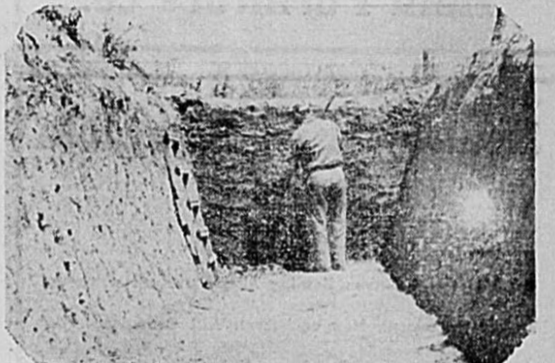
A development of the past few years has been the storage of whole grain in trench silos.
