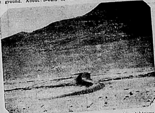
Spreader dam on the Otis Kimball ranch, Brewster county. The structure catches run-off water in the creek and throws it out on the grass flats on either side and below the dam.
