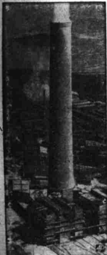
BOLT TRAP —Copper spikes top 585-foot-high stack at Anaconda Copper Mining Co., Anaconda, Mont., to coax lightning down shaft to measure intensity and duration.
