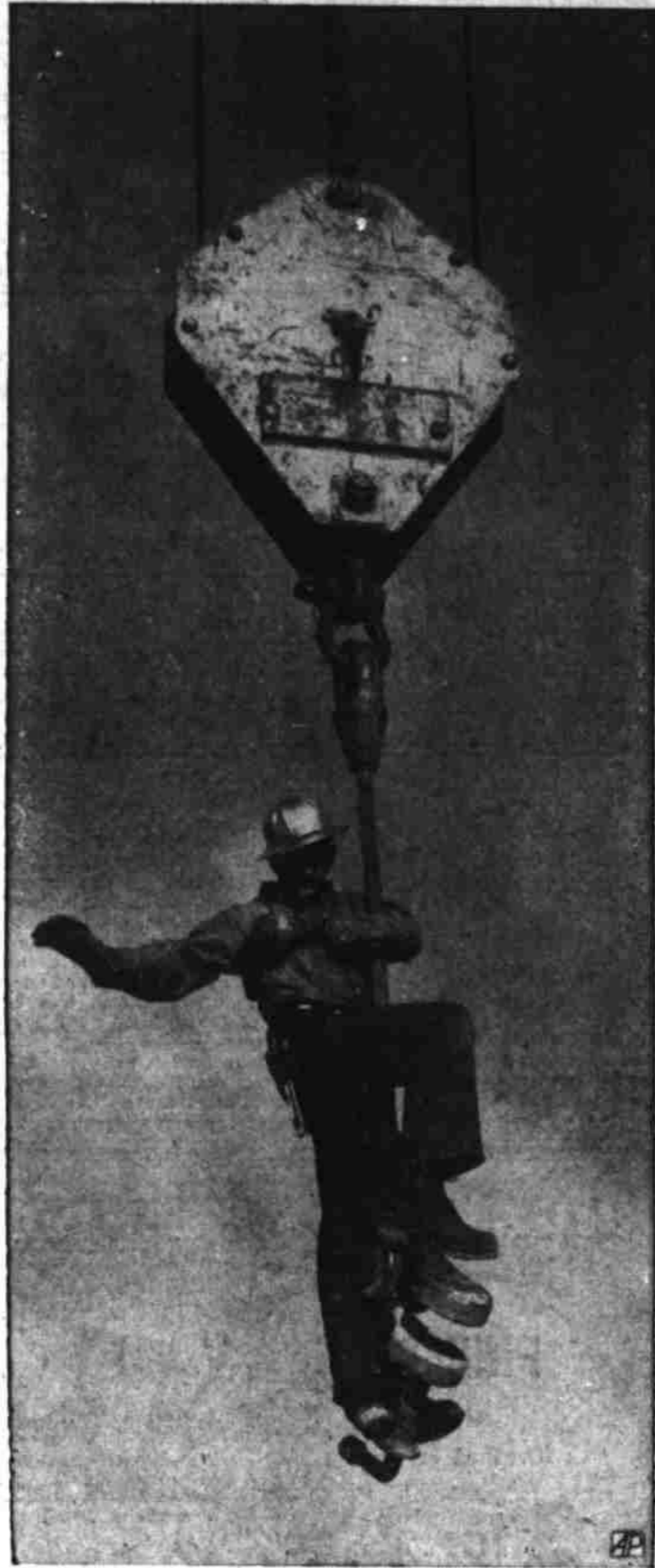
AERIAL ELEVATOR —There's no stopping for floors when a construction worker at the Friant dam being built on the San Joaquin river near Fresno, Cal., descends. This fellow rides the hook of a traveling crane being maneuvered to pick up a load.
