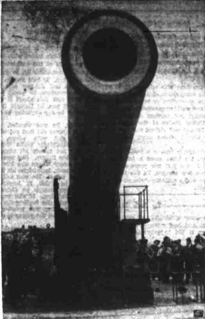
SLEEPING BEAUTY—This big 16-inch coast defense gun at Fort Tilden, N. Y., hadn't been fired in five years until America suddenly became defense-conscious. It shoots half-ton shell nearly 17 miles. The new defense program earmarks $250,000,000 for arms plant expansion, $200,000,000 for munitions tools, $30,000,000 for manufacture of new anti-aircraft gun.
