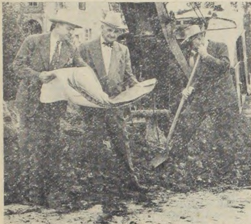
CONSTRUCTION BEGINS—Pres. D. M. Wiggins, right, is shown recently as he breaks ground for the addition of two wings to the Administration building. W. G. McMillan, contractor, left, and W. T. Gaston, college business manager study the plans for the construction.
