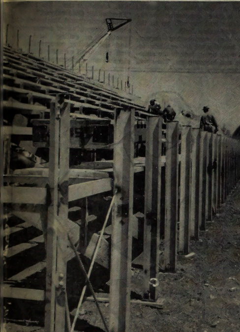
NEW SEATING FACILITIES NEARING COMPLETION
