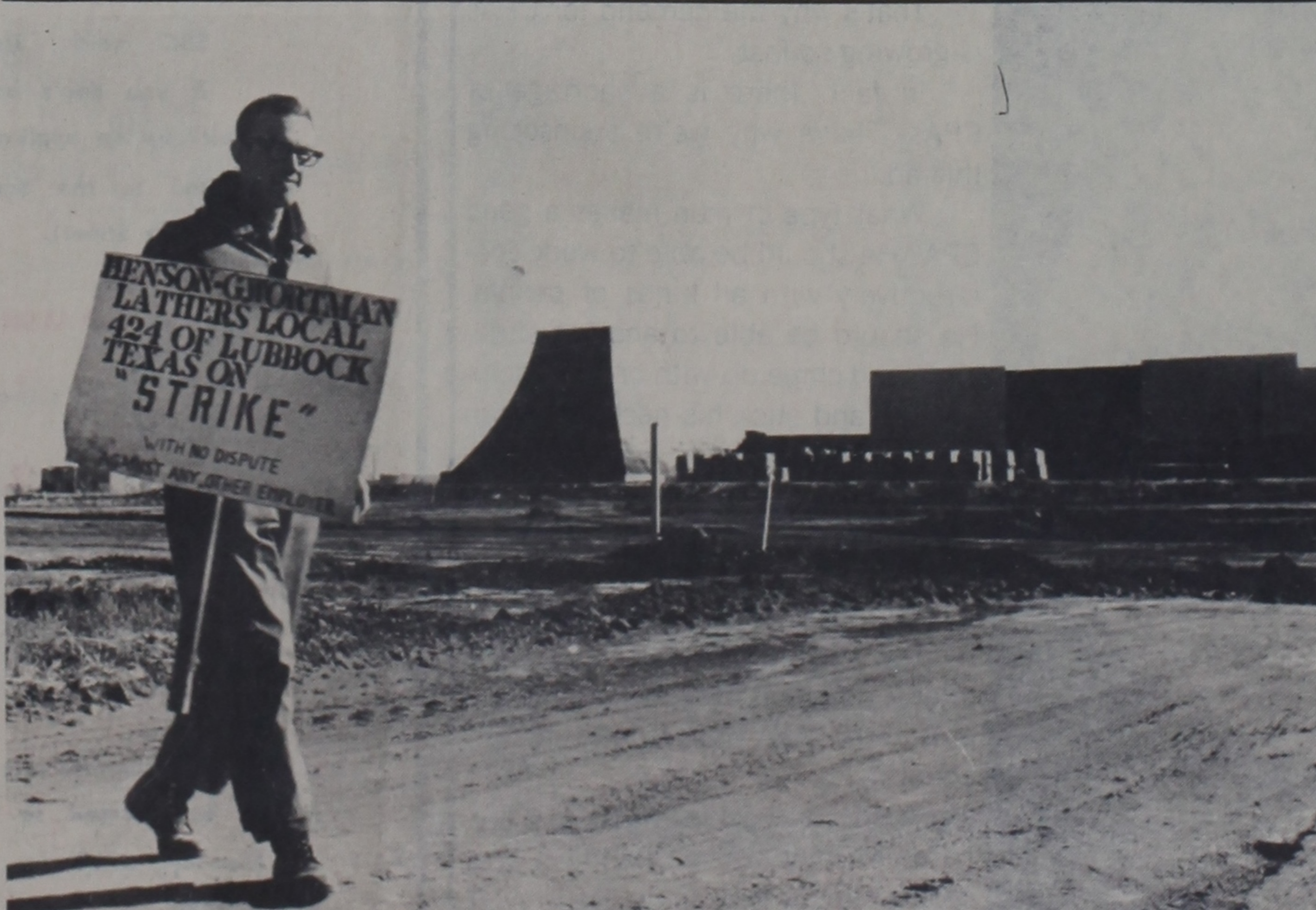
MUSEUM STRIKE—The Lathers Union strike which is holding up work on the West Texas Museum carried into the tenth day yesterday as a lone picket walked near the construction site. Contractor and Union representatives did not meet yesterday. Ralph
