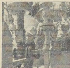
**MAINTENANCE TEAM** making a speedy change of a methanol valve to minimize production loss.
