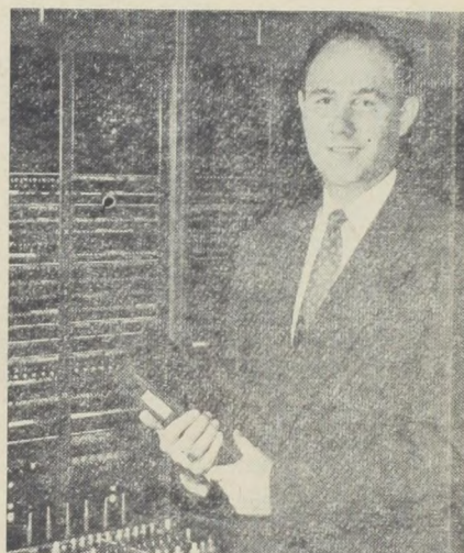
Emmett Smith supervises operation of this training switchboard, which he originally helped to design.
