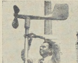
Carl Gosline, B.S., Iowa '41, conducts meteorological engineering studies to help solve plant chimney problems involving smoke and acids.
