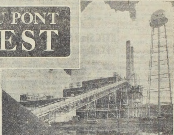
This powerhouse for a nylon plant at Martinsville, Va., was designed by Dr. Pont engineers. It houses two 135,000 lb./hr. boilers and two 7,500 KW extraction turbine generators.
