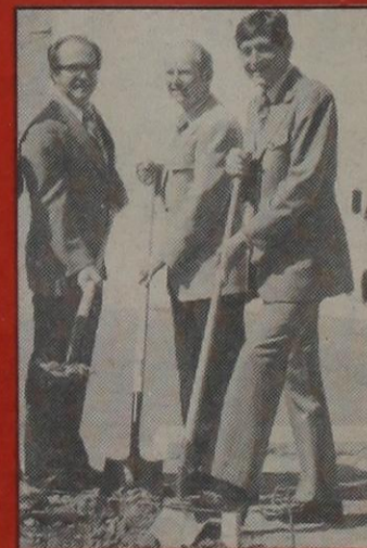
Shown here during ground breaking for the latest Varsity expansion which included the addition of the 13th street entrance are l to r: Chester Banks, Dave Andrews and W. B. (Dub) Rushing.
