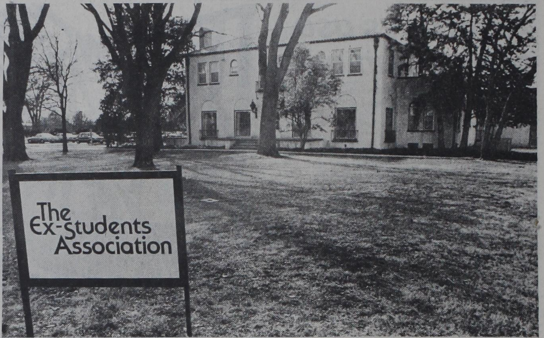
This building, near the southeast corner of the campus, houses the Tech Ex-Students Association. (Photo by Max Faulkner)
