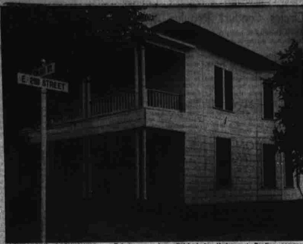
ATTRACTIVE REFINISHING — Exteriors can be refinished by Underwood Roofing company to give the attractive appearance of a new building. Here is a typical example where asphalt siding, expertly installed, transformed the appearance of a home. Of course, the Underwood service extends to various types of conventional and special roofing. Those of fire-proof qualities are a specialty. (Jack M. Haynes Photo)
