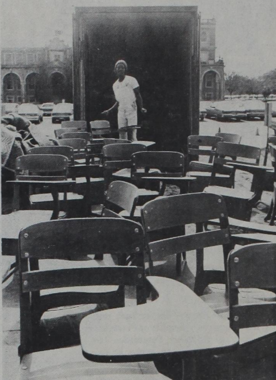
Outdoor class? Taking a break for the camera, Ronny Davis moves new desks into the Social Science Building. The building is undergoing renovation and will eventually house the mathematics department. (Photo by Ted Houghton)
