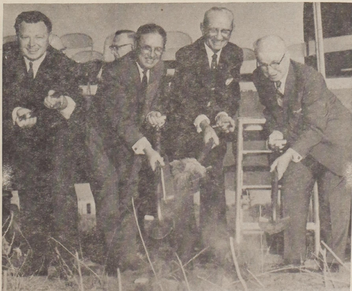
NEW DORM STARTS OFF IN A CLOUD OF DUST —Four dignitaries dig in during ground-breaking ceremonies for the new men's dorm to be built in the 1500 block on Orlando west of the campus. Left to right, Robert Colglazier, vice-
