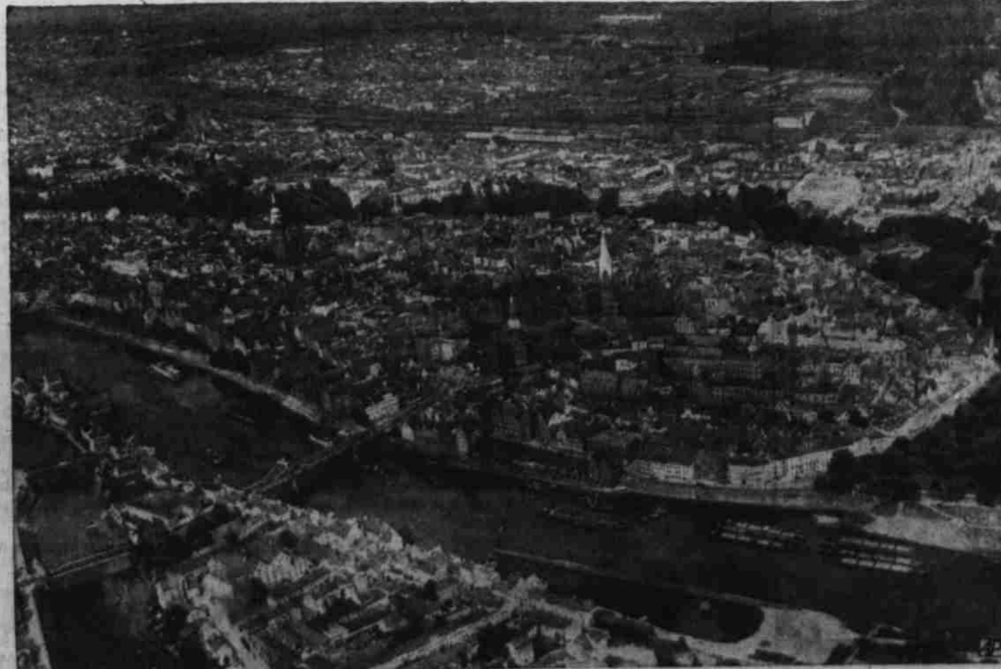
FEELS ALLIED BOMBING FURY —Allied bombers have struck many times at Bremen, German seaport and industrial city on the North Sea, with the city's aircraft plants as their special target. This aerial view was made before the war.
