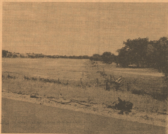
Fence, Silt and Scour Damage
