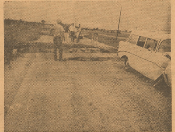
Bridge Washout On Farm To Market Road East of Carbon In Kokomo Community During Floods Of June 10, 1967.
