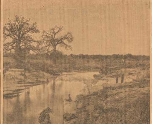
Uncontrolled Floods Are Expensive — This bridge had to be replaced completely by the county. It was washed out as a result of flooding in September of 1964. The picture was taken north of Duster on the county road a short distance east from W. M. Haynes' home. Mr. Haynes can be seen in the background repairing fence that was also washed out during the same flood.
