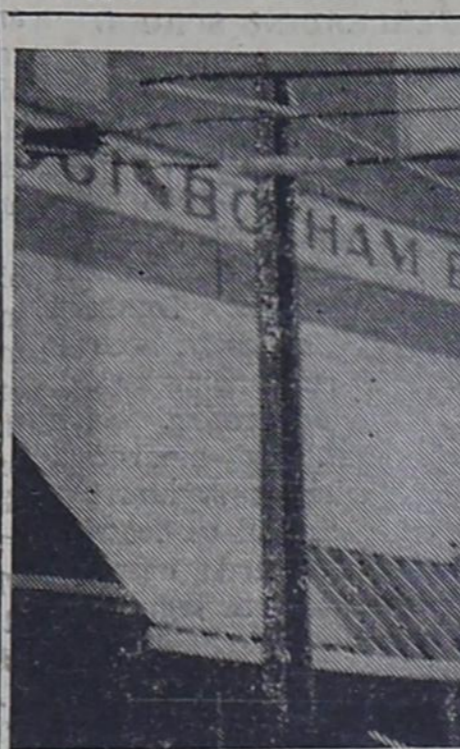
HIGGINBOTHAM'S GET NEW FACE LIFT — Higginbotham's is remodeling the front of their store with a new awning and will install new glass doors on the front. Much of the floor space inside has been repaired with new cement and other remodeling projects are underway.
