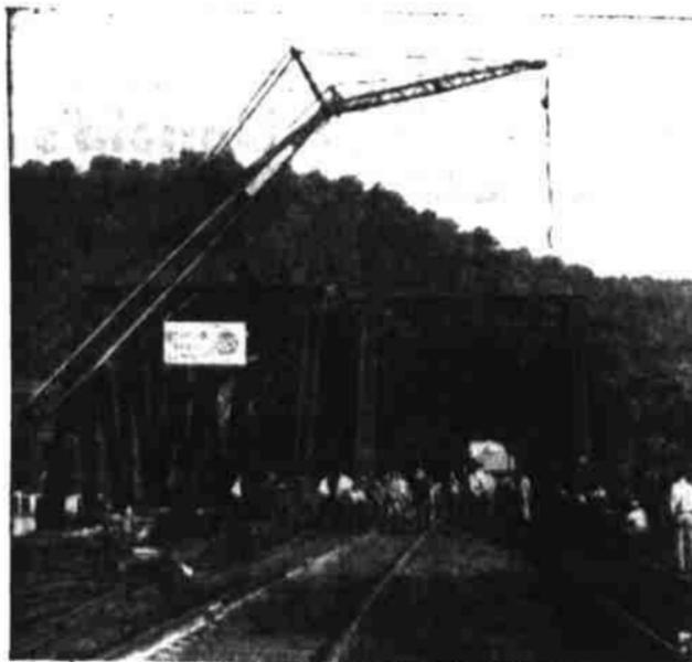
BRIDGE SUPPLANTS BRIDGE —A Pennsylvania Railroad bridge at Warren, Pa., (right) is moved from its piers onto temporary piling while a new bridge (left) is rolled into its place by a winch that controls cables of both.
