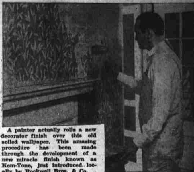
A painter actually rolls a new decorator finish over this old soiled wallpaper. This amazing procedure has been made through the development of a new miracle finish known as Kem-Tone, just introduced locally by Rockwell Bros. & Co.
