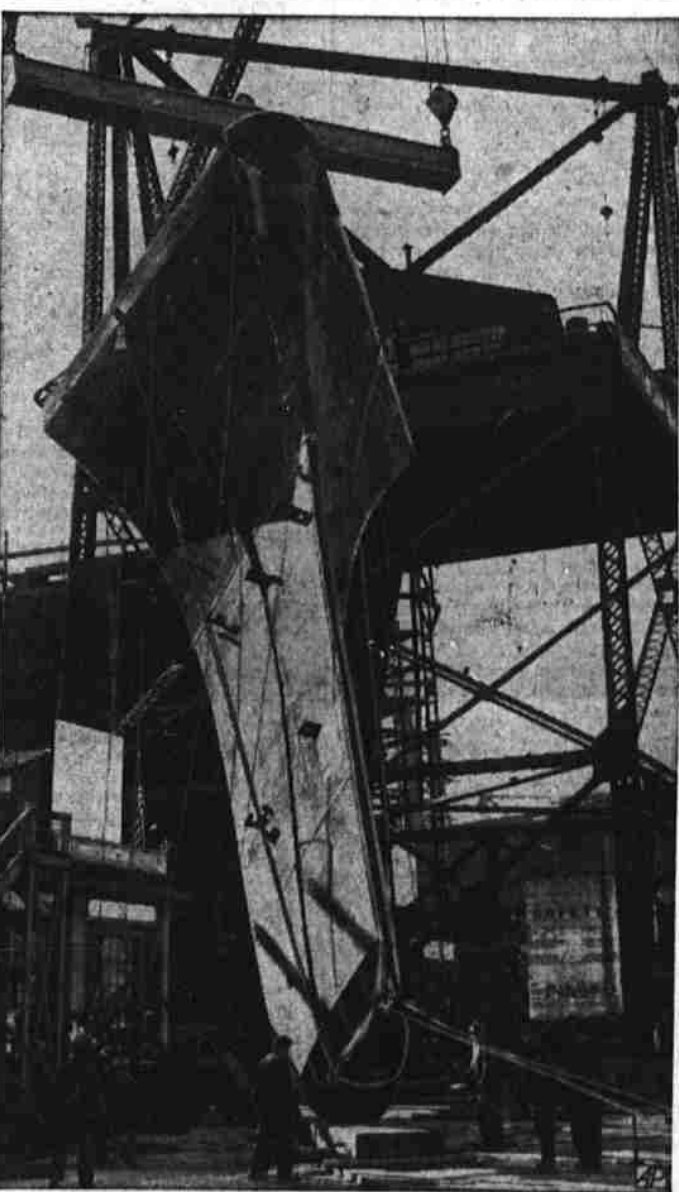
NOSE FOR A SHIP—Sixty feet tall and weighing 100,000 pounds, this bow of a cargo ship is carried by a crane to a half mile away where it will be fitted to a hull under construction at Federal shipyards, Kearny, N. J.
